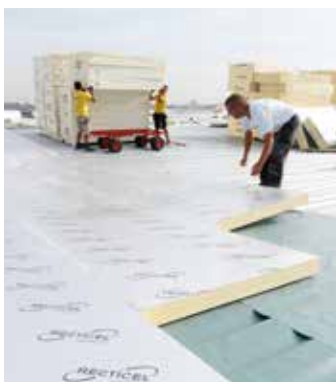
Roof insulation (flat and pitched roofs)
